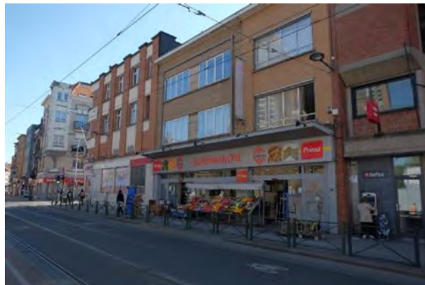
Figure 102 : Constructions longeant la chaussée de Helmet (ARIES, 2020)
